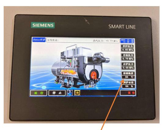
Operation data: Exhaust gas temperature 55°C
